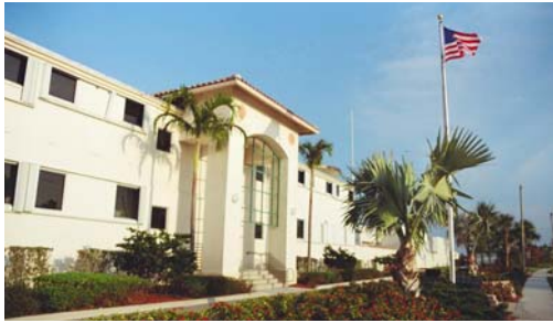
East Water Treatment Plant
